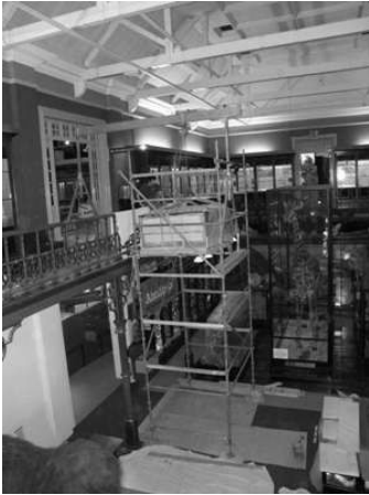
Kiln coming over the Balcony
