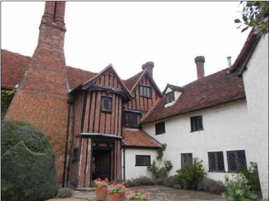
Originally the back entrance, this is now the front door
