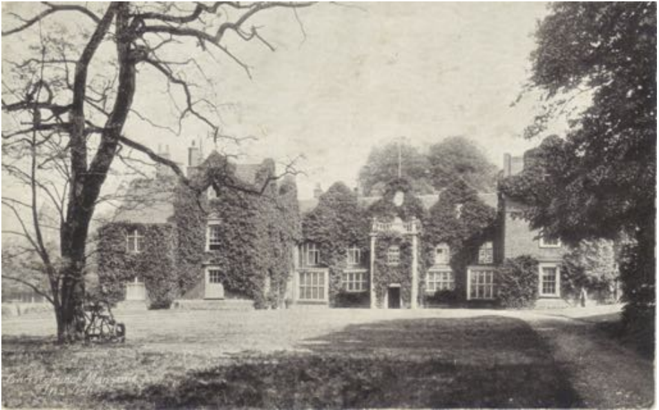
The ivy-clad Mansion
